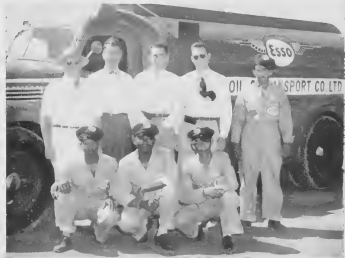
Here are the men who made the refueling operation successful. Standing, left to right: N. L. Holland, L.O.F., who will supervise the field crew; J. H. Wukbold, Esso Marketing representative, N.W.I.; Ed Gavin, who advised on the operation of equipment and supervised the safety features required; W. L. Kaestner, Marketing assistant; and Jaente Rosell-Kneeling; Alford St. Louis, Magnus Billy, and Guillermo Tromp.
